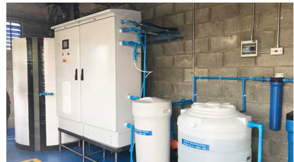
Finanalyte FIN 1800HD set for 5000ppm for public water treatment
